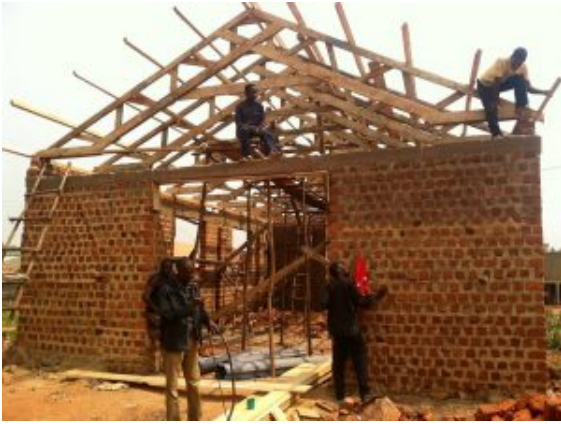
Roof rafters built on the site and lifted and raised into their position to hold the roofing
