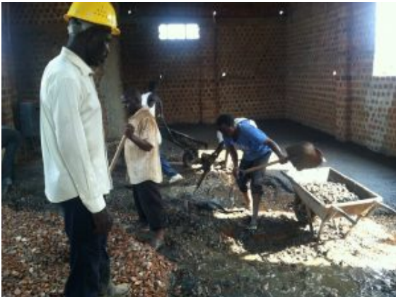
From the outside to the inside. Construction Engineer, Pastor Sande Toto oversees the pouring of the cement floors in early January 2018.
