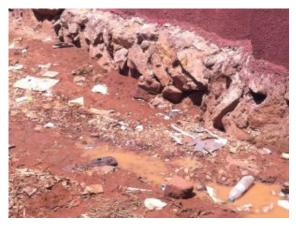
The water damage that the flooding rains had caused to the foundation of the Milling Project's newly built building in Kiereka Kasokoso.
